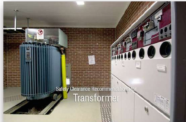
TRANSFORM DG CLEARING
