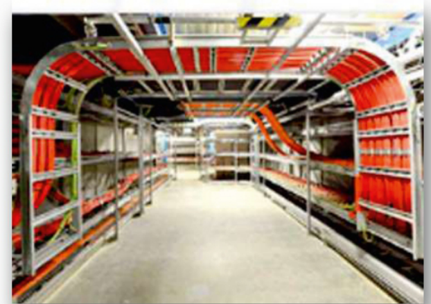
Cable Tray Installation
