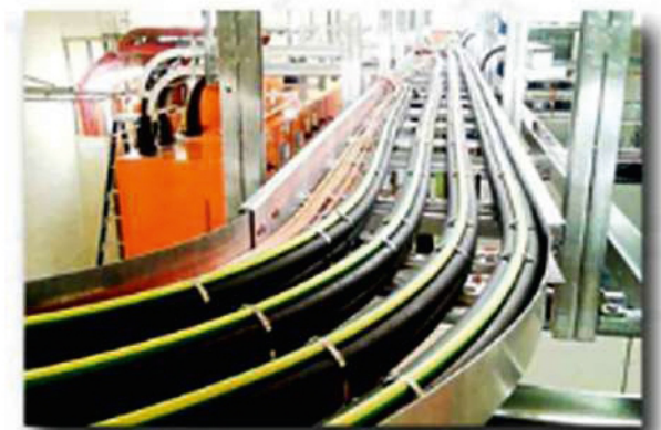
LT/HT Cable Laying
